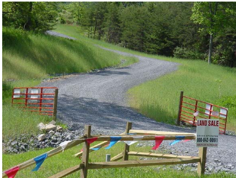
Figure 2.2: New Subdivision in Hampshire County. Photo by David Warner.
